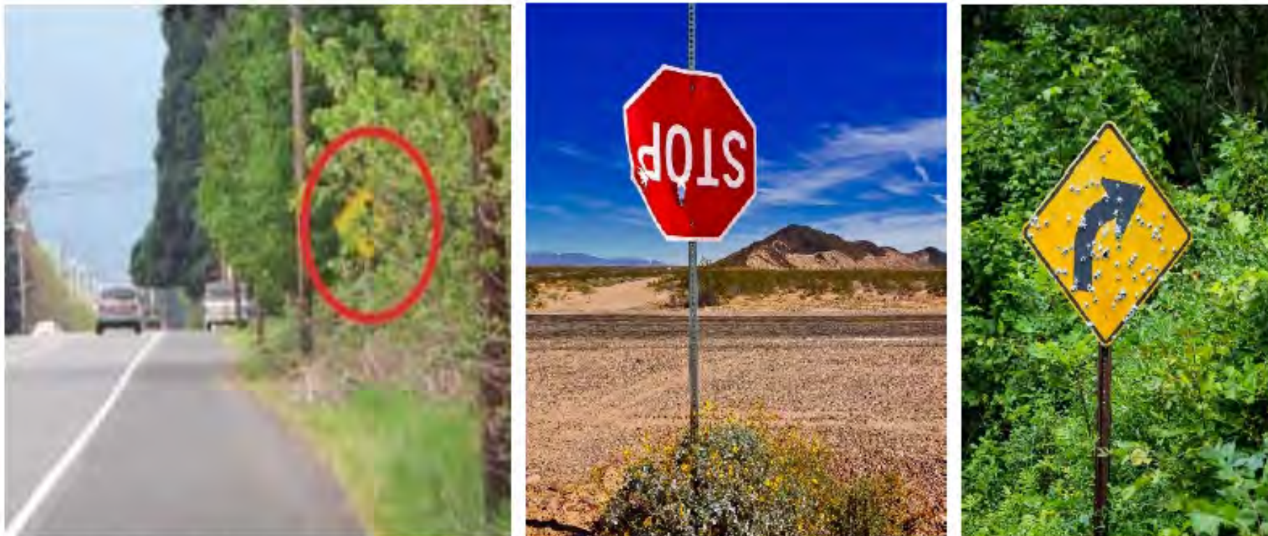
Figure 3-6. Examples of problematic signage with sign blocked (left) and damaged signs (right)
