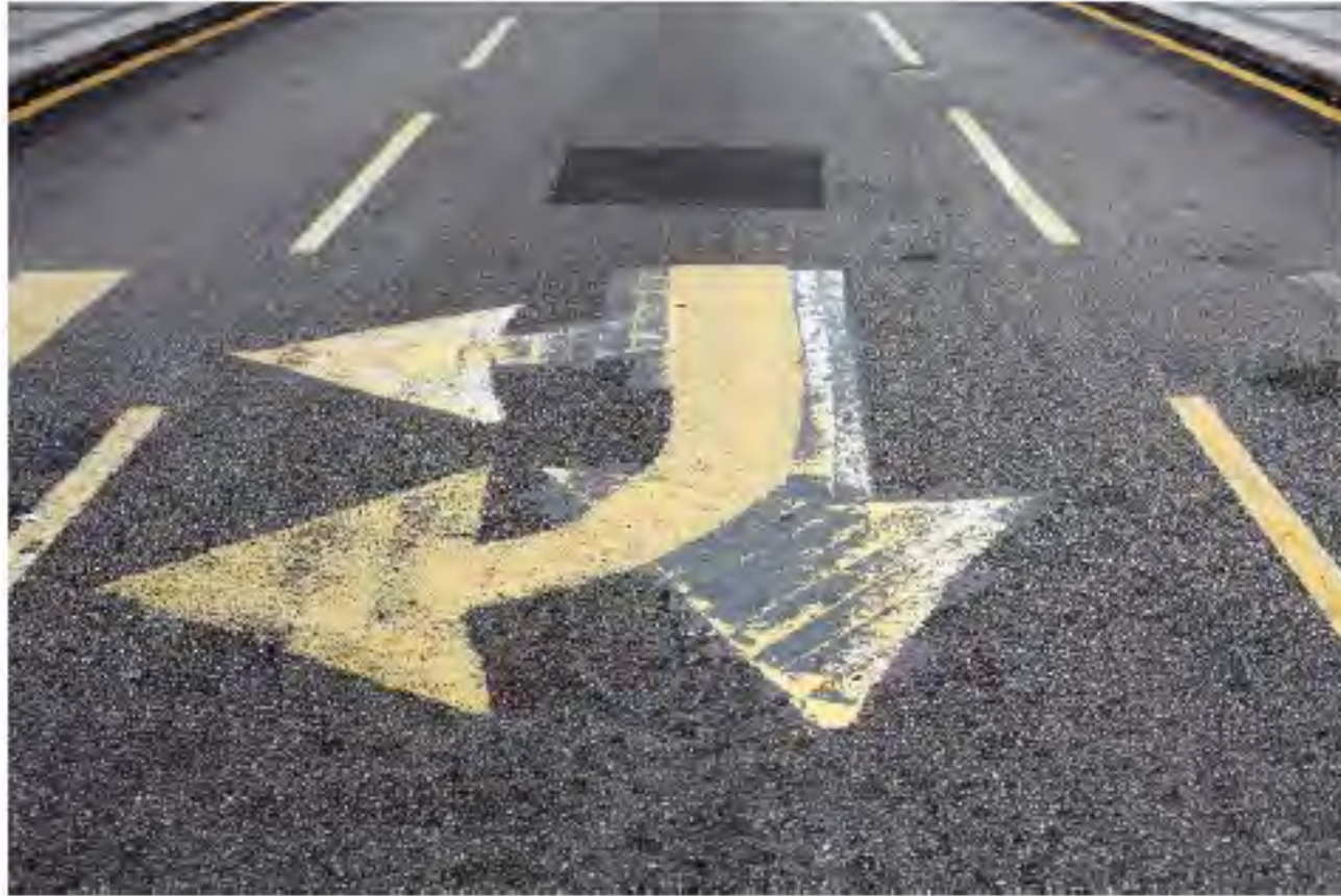
Figure 3-2. Example of overlapping pavement markings
